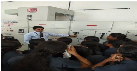
Students at Field Visit – “RIT Power House”
