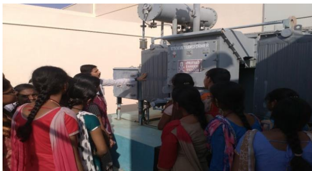
Students at Field Visit – “RIT Power House”
