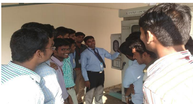
Students at Field Visit – “RIT Power House”
